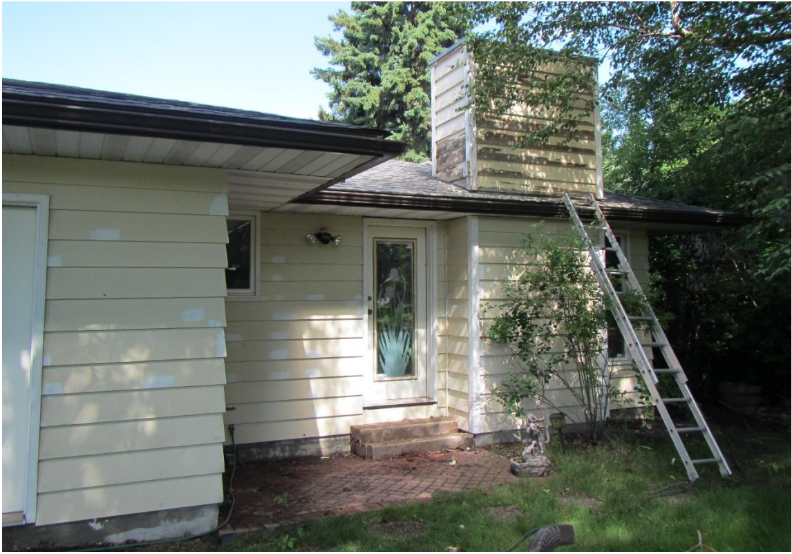
EXTERIOR PAINTING – Wood Siding and Window/Doorframes – BEFORE
